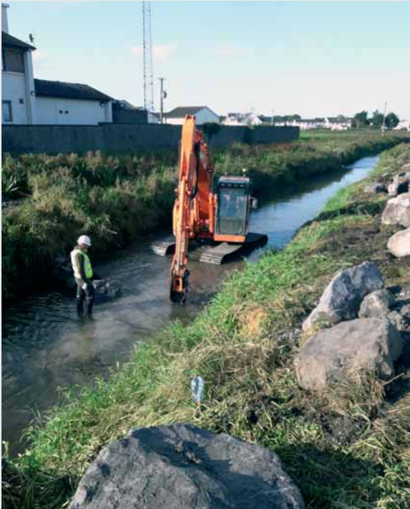
Excavation of a pool in the Nanny River in Tuam.
